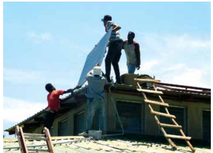
Installing the solar panels for the Library.
